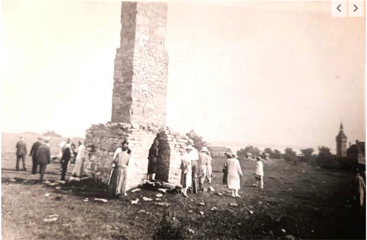
The Jefferson County Historical Society hosted a trip to Carleton Island in July 1926. This group explores chimney remnants of Fort Haldimand. The building sphere in the background on the right is a 111-foot high tower that was separate from Carleton Villa. "A brilliant gas light, long illuminated in the tower, became a range beacon for navigators passing down the American channel before the government protected the shoal off the head of the island by a light buoy," the Watertown Daily Times reported. Watertown Daily Times
