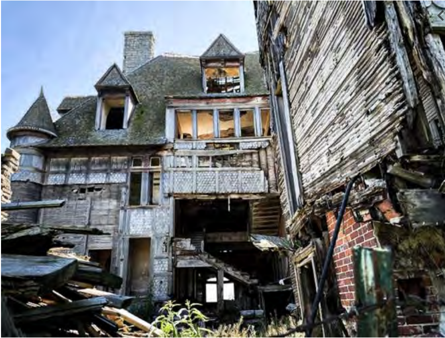
The deterioration of the villa on Carleton Island. Contributed.
