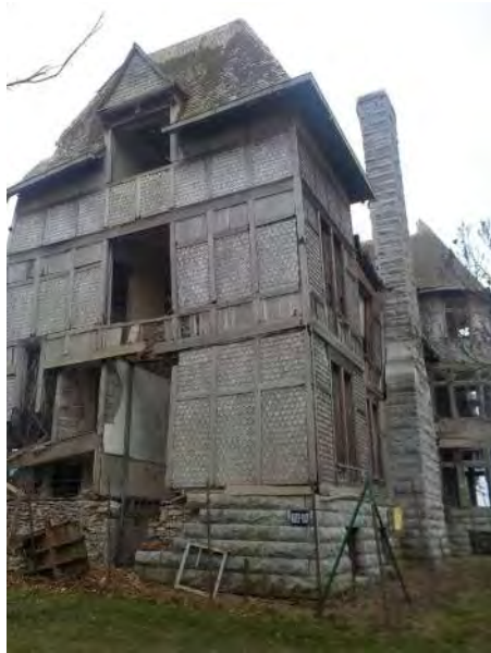
063 - Northeast Area - North corner 1.jpg
