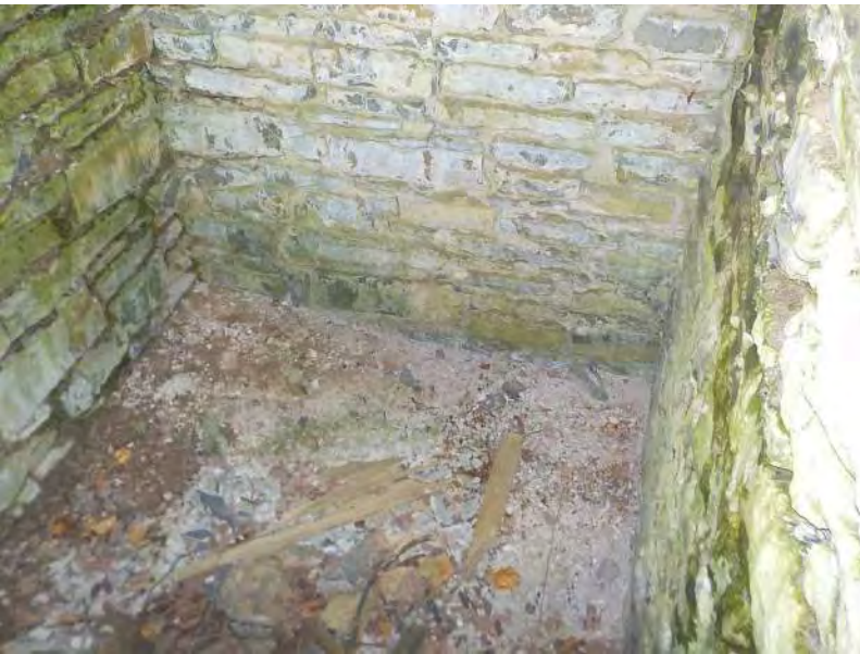
033 - Exterior masonry - Vault under SW entrance.jpg
