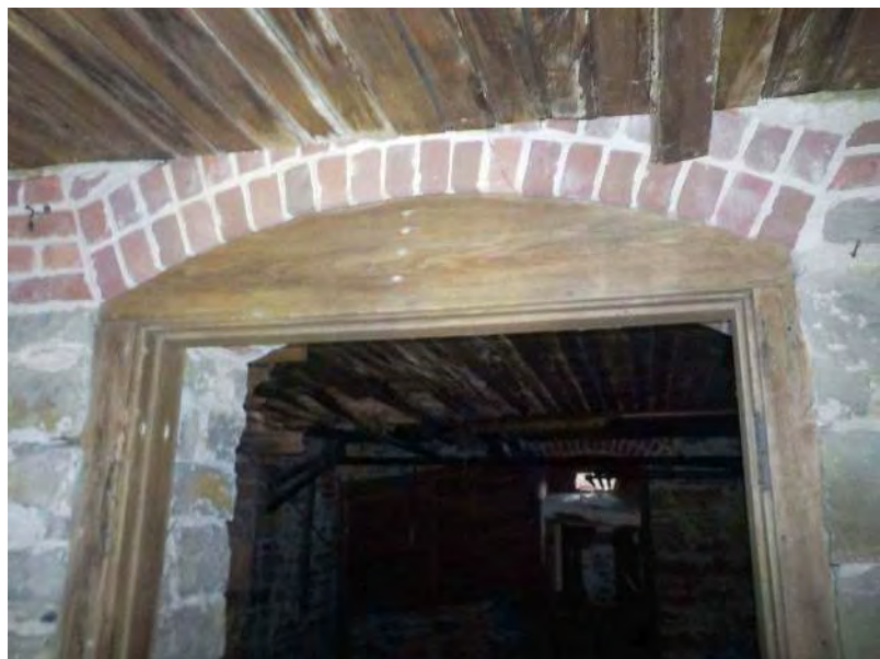
150 - Basement - Arch over opening 5.jpg
