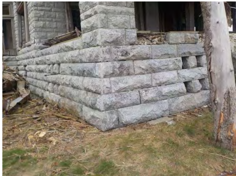
042 - Exterior masonry - Cut stone at perimeter walls.jpg
