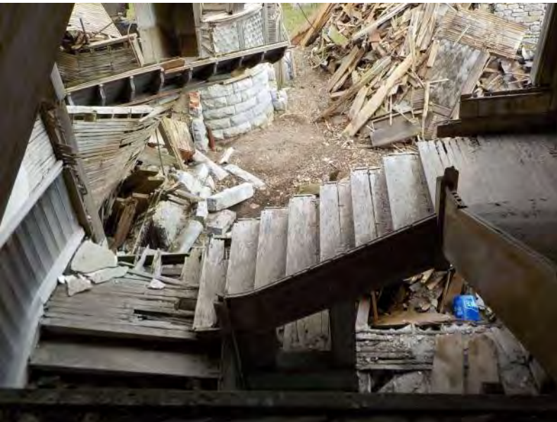
093 - Third Floor - Looking down staircase.jpg
