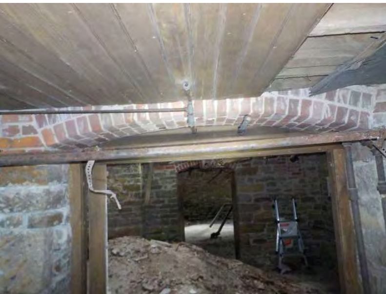
151 - Basement - Arch over opening 6.jpg
