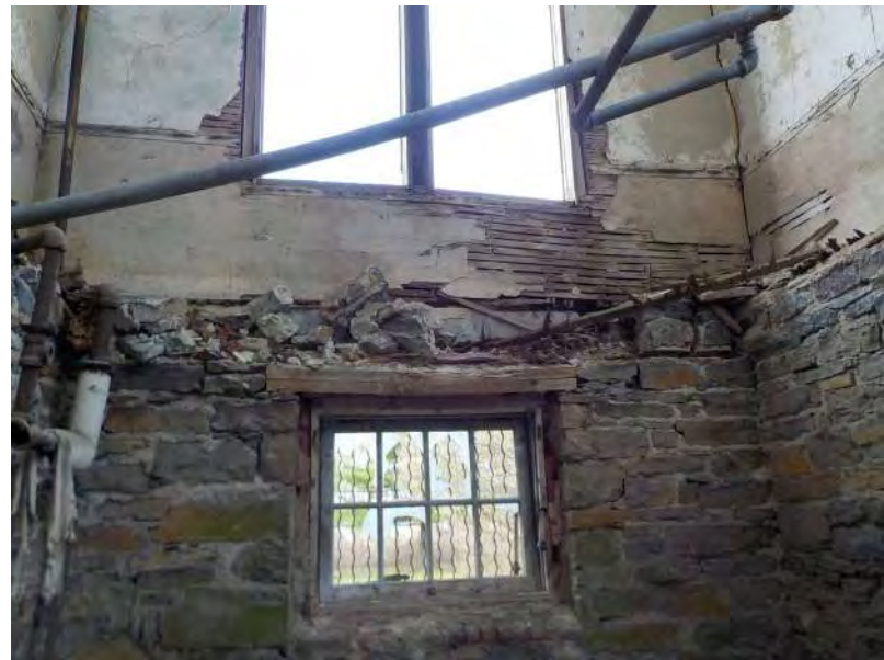
072 - Northeast Area - Inside face of basement wall.jpg
