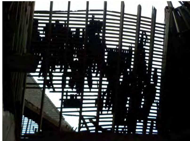
084 - Third Floor - Looking up at roof framing 3.jpg
