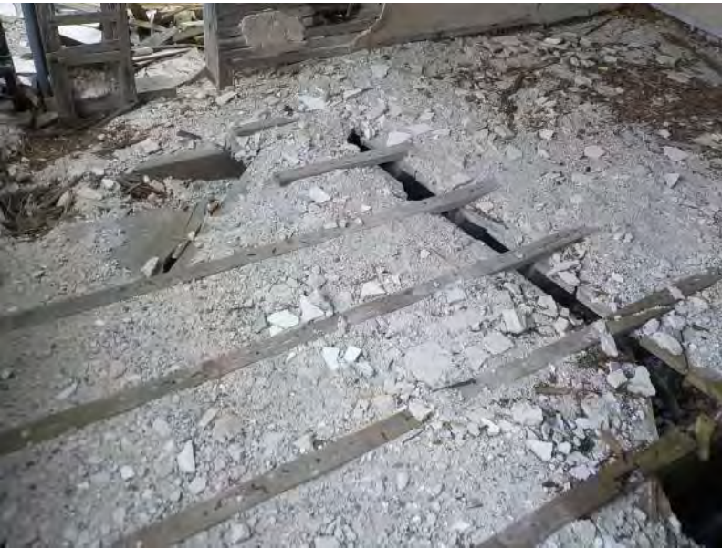
109 - Second Floor - Overview of floor 4.jpg
