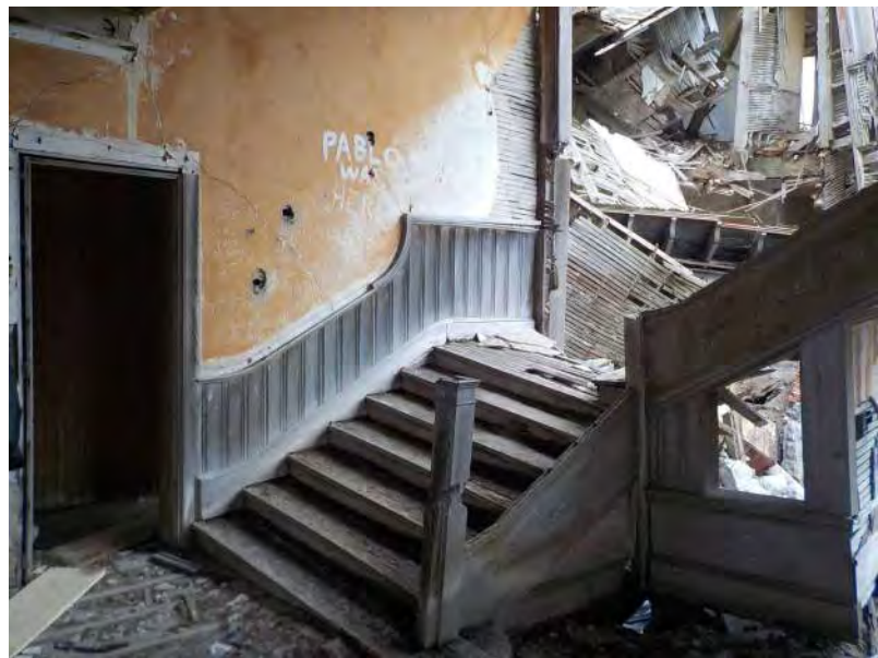
116 - First floor main staircase 1.jpg
