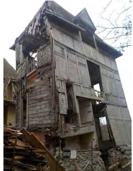
064 - Northeast Area - North corner 2.jpg
