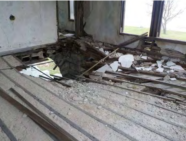
111 - Second Floor - Overview of floor 6.jpg
