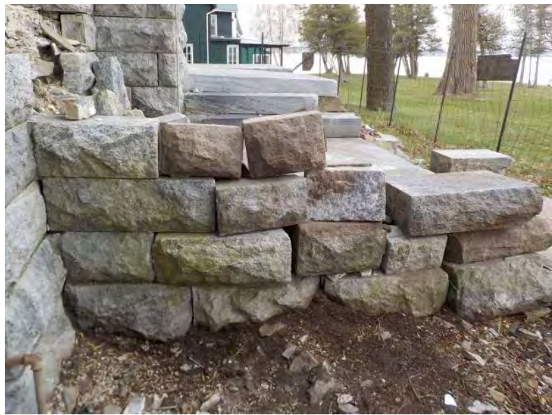
032 - Exterior masonry - SW entrance 8.jpg
