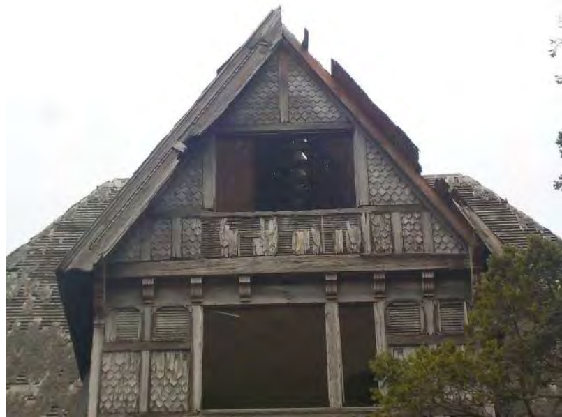
010 - Upper building exterior overview 4.jpg
