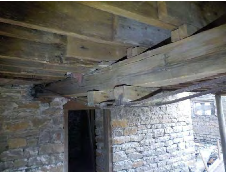
141 - Basement - First floor kingpost beam 1.jpg
