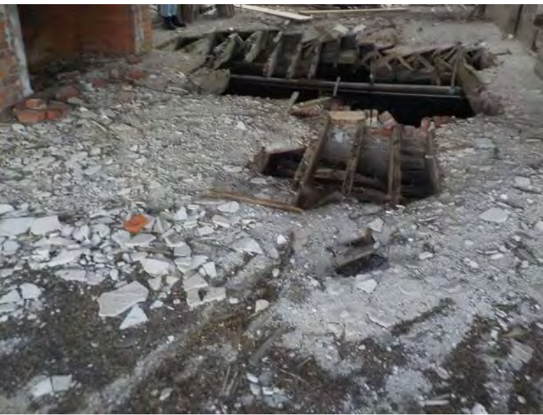
133 - First Floor - Overview of floor 7.jpg
