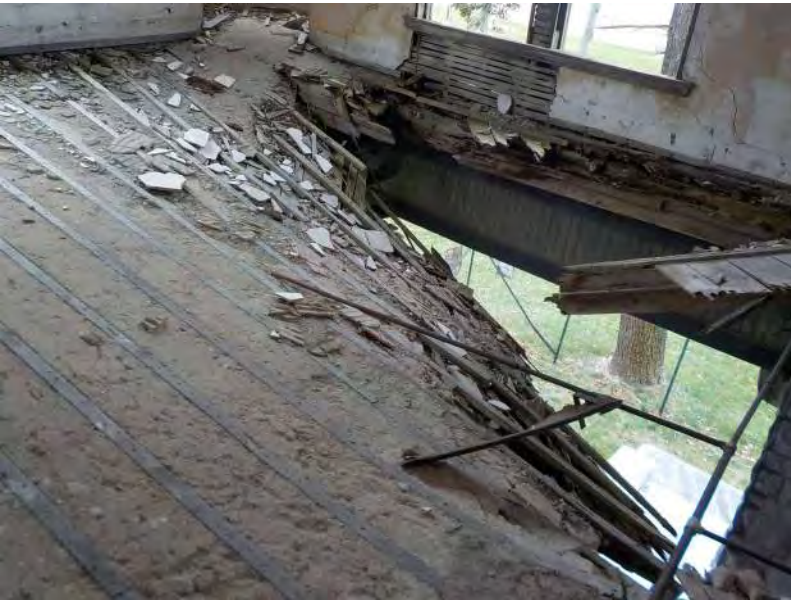
113 - Second Floor - Overview of floor 8.jpg
