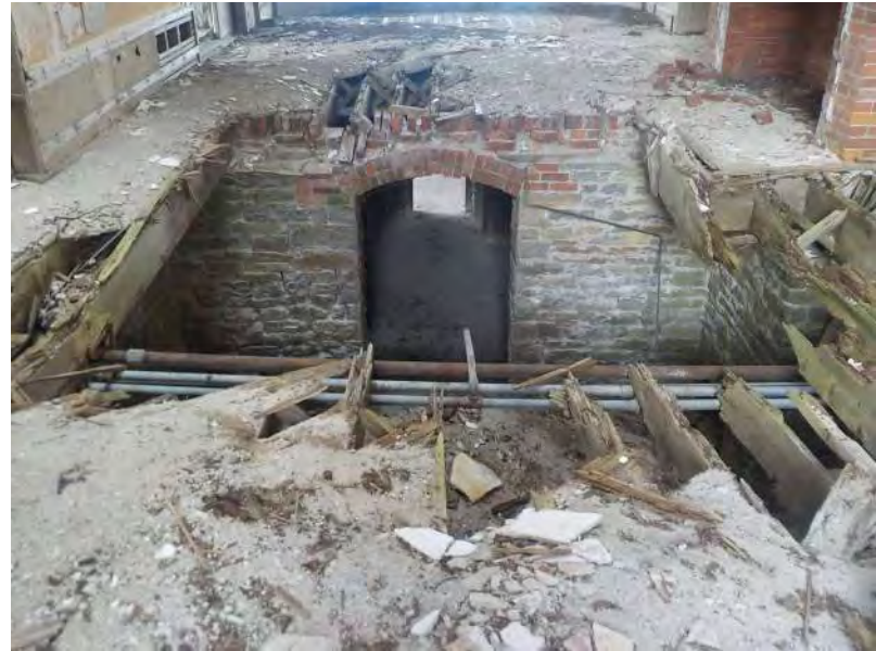
130 - First Floor - Overview of floor 4.jpg
