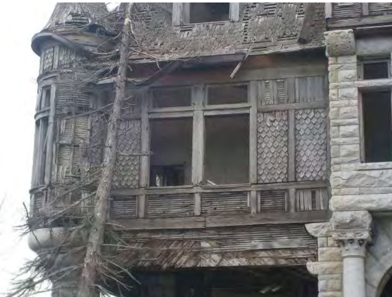
011 - Upper building exterior overview 5.jpg
