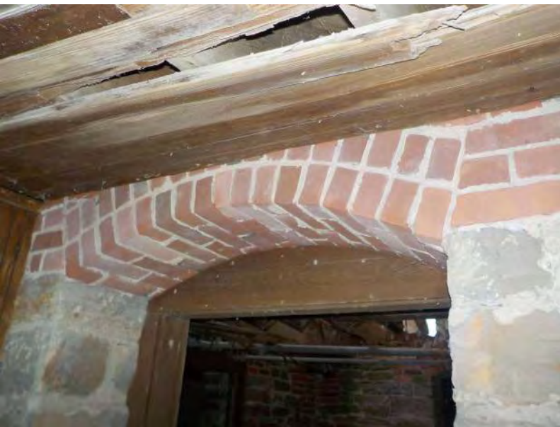
145 - Basement - Arch over opening 1.jpg
