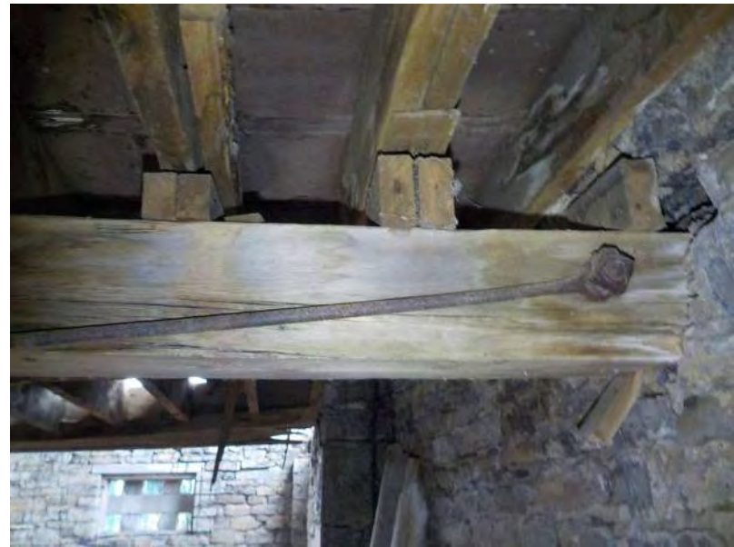
142 - Basement - First floor kingpost beam 2.jpg
