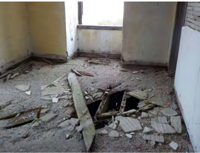
091 - Third Floor - Overview of floor 1.jpg
