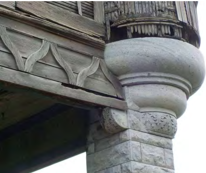
039 - Exterior Masonry - Stone turret at south corner.jpg
