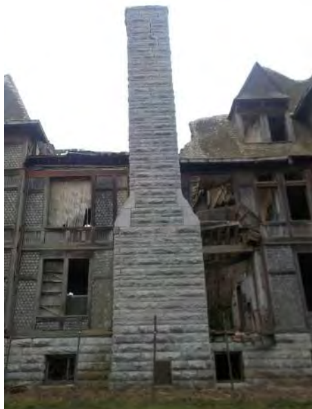
077 - Northeast Area - Chimney NW face.jpg
