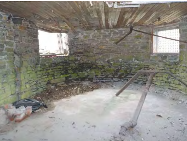
143 - Basement - Overview of stone walls from interior 1.jpg
