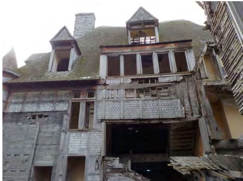
016 - Upper building exterior overview 11.jpg
