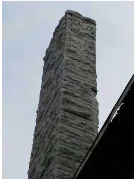
081 - Northeast Area - Chimney SW side.jpg
