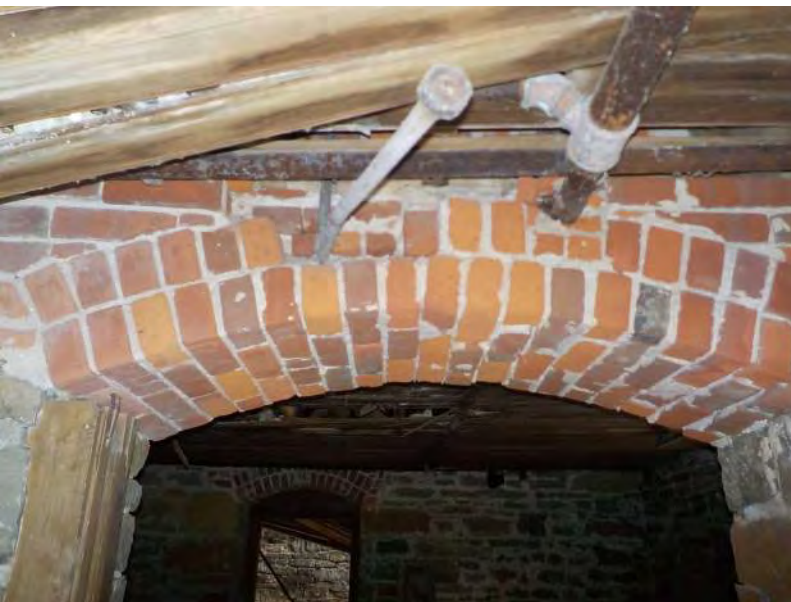
147 - Basement - Arch over opening 3.jpg
