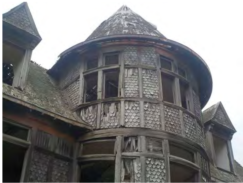
008 - Upper building exterior overview 2.jpg
