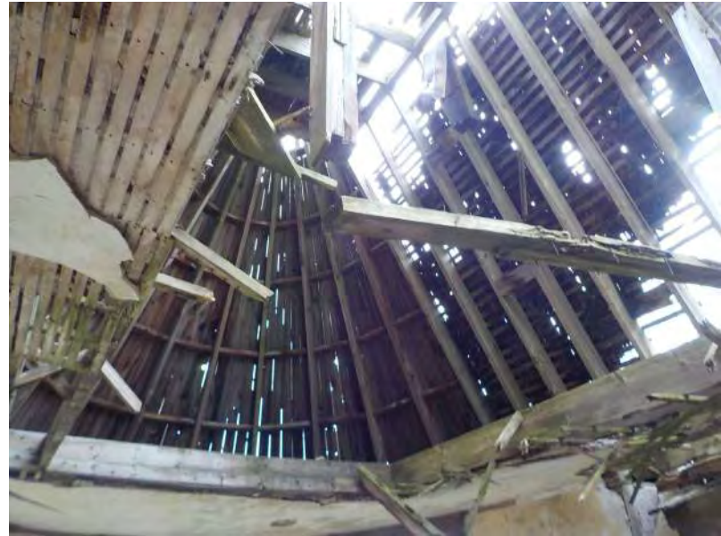
082 - Third Floor - Looking up at roof framing 1.jpg
