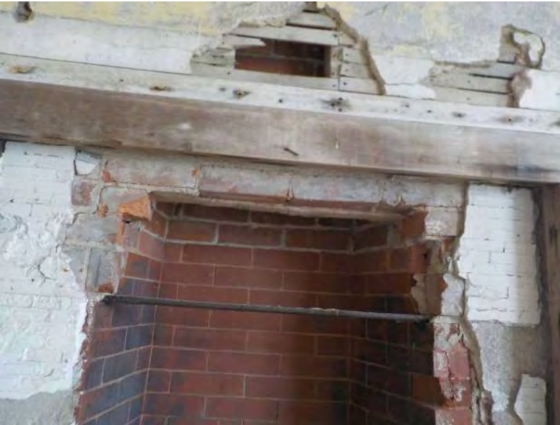
105 - Second Floor - Fireplace 2.jpg
