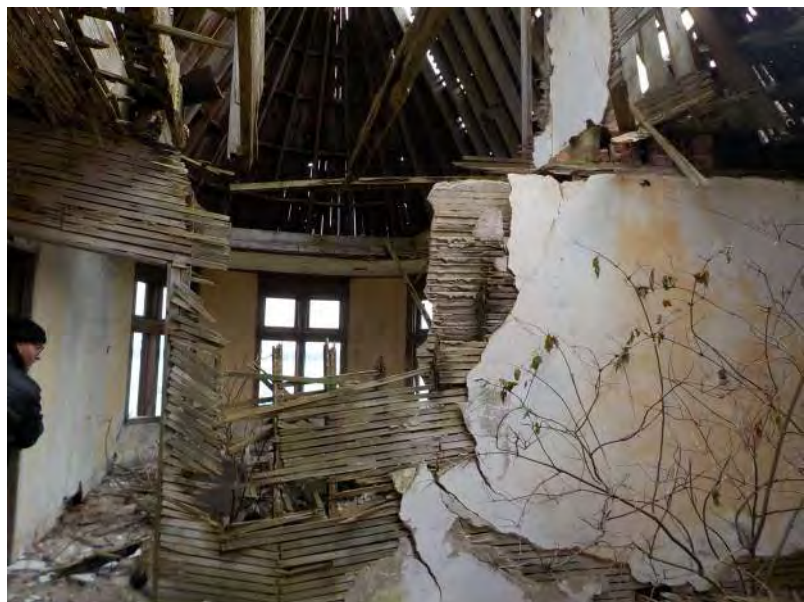
090 -Third Floor - Interior partitions.jpg
