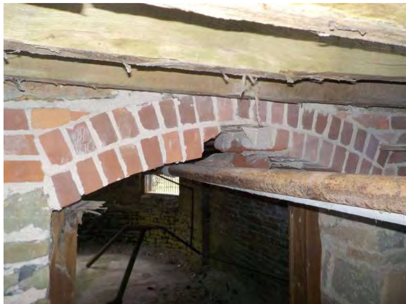
146 - Basement - Arch over opening 2.jpg
