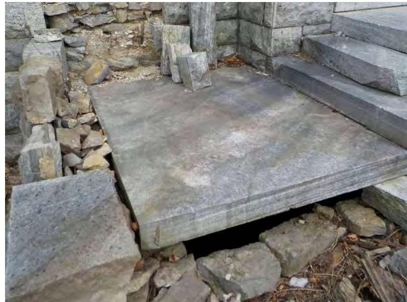
028 - Exterior masonry - SW entrance 4.jpg
