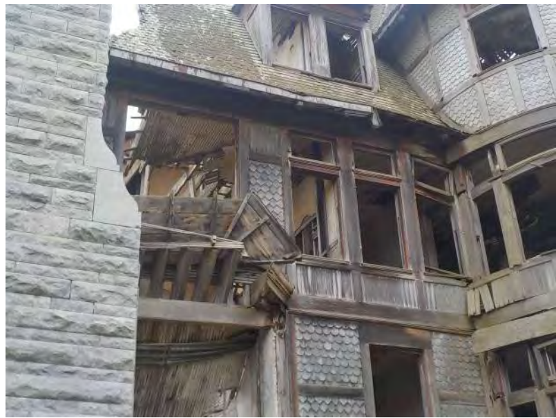
014 - Upper building exterior overview 9.jpg
