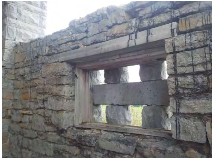
154 - Basement - Wood plank lintel over opening 3.jpg
