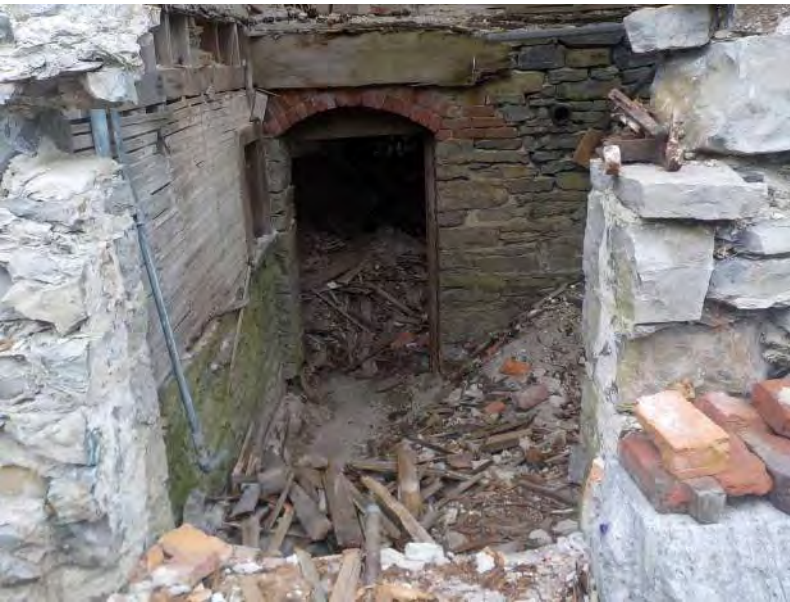
069 - Northeast Area - Basement walls 1.jpg
