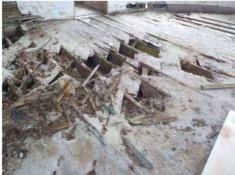
108 - Second Floor - Overview of floor 3.jpg
