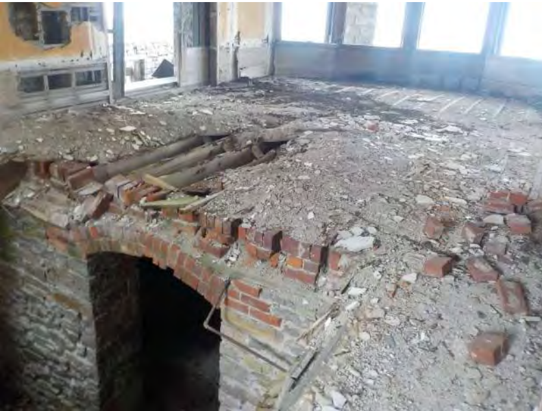
131 - First Floor - Overview of floor 5.jpg
