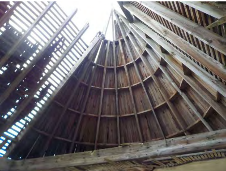
083 - Third Floor - Looking up at roof framing 2.jpg
