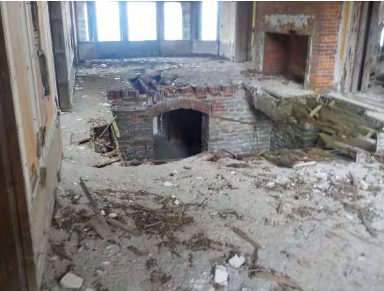
129 - First Floor - Overview of floor 3.jpg
