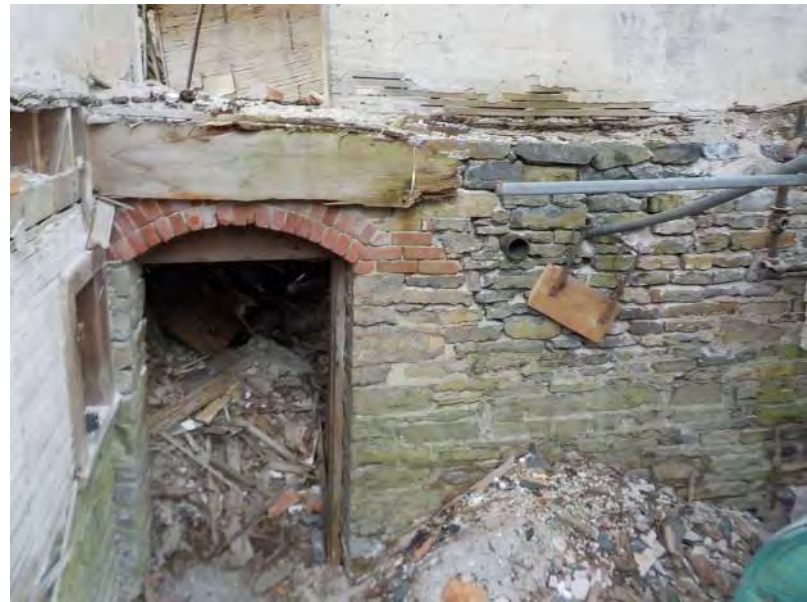
070 - Northeast Area - Basement walls 2.jpg
