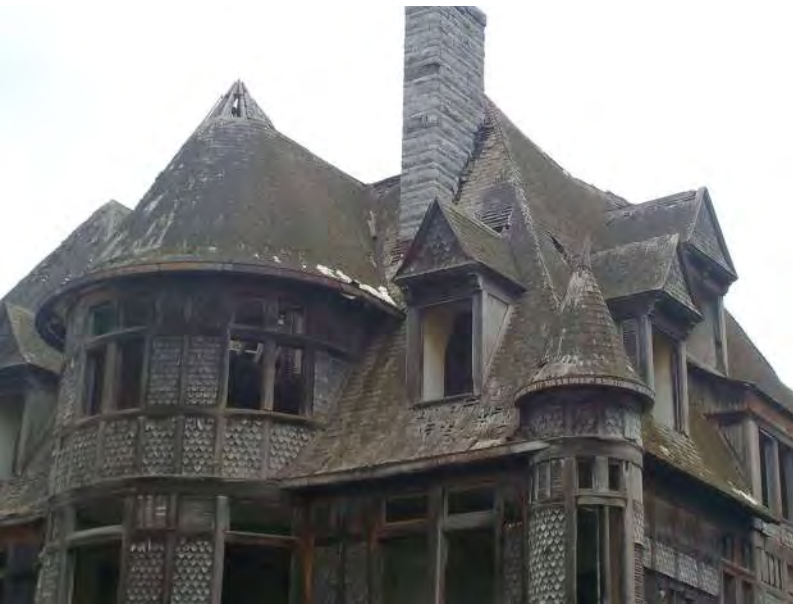
007 - Upper building exterior overview 1.jpg
