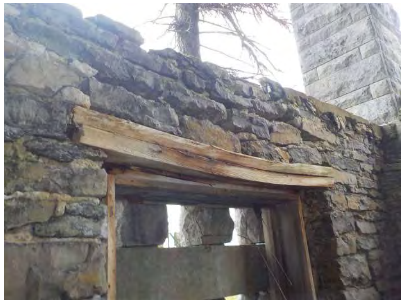
152 - Basement - Wood plank lintel over opening 1.jpg
