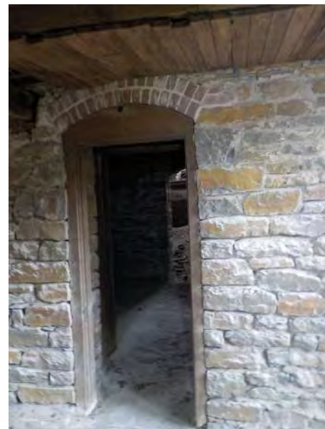
148 - Basement wall and opening arch 3.jpg
