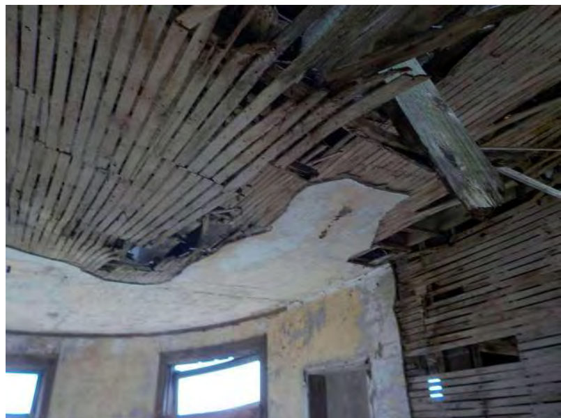
096 - Second Floor - Overview of ceiling.jpg
