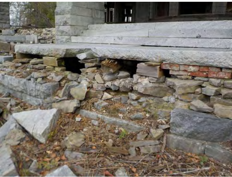
031 - Exterior masonry - SW entrance 7.jpg
