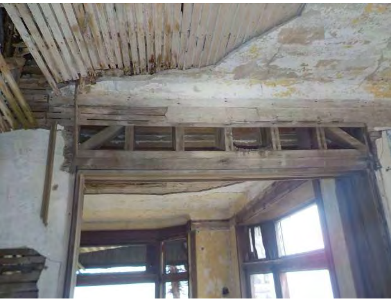
121 - First Floor - Wall opening header 12.jpg
