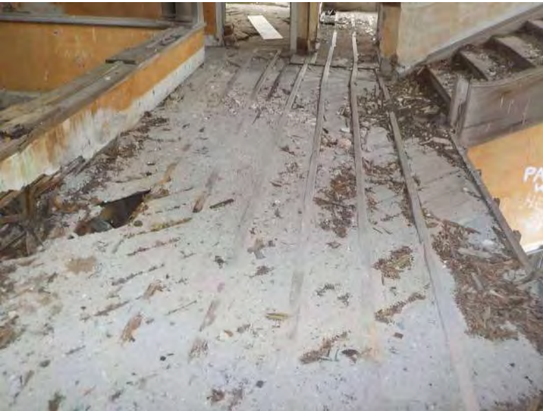
107 - Second Floor - Overview of floor 1.jpg
