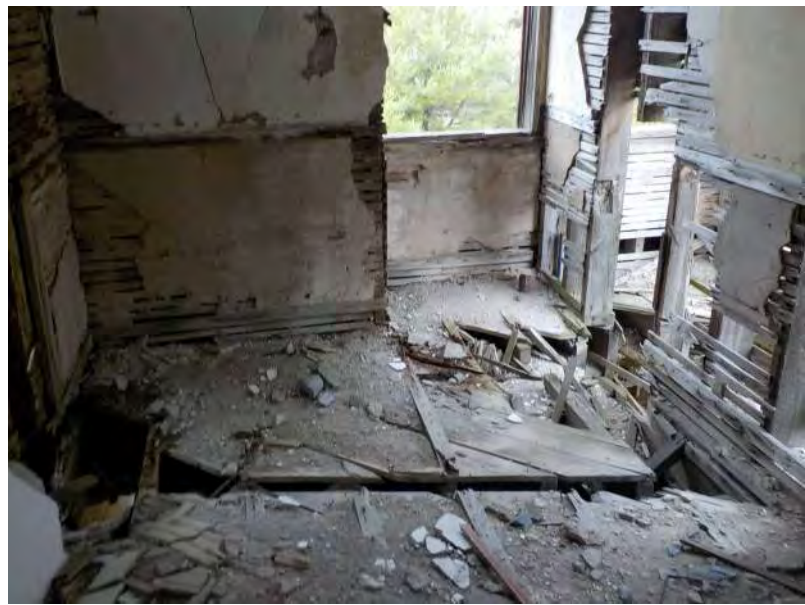
092 - Third Floor - Overview of floor 2.jpg
