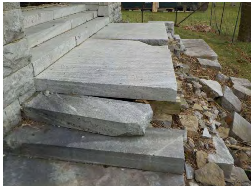
030 - Exterior masonry - SW entrance 6.jpg
