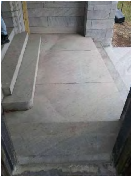
035 - Exterior - Stone stoop at SE entry.jpg
