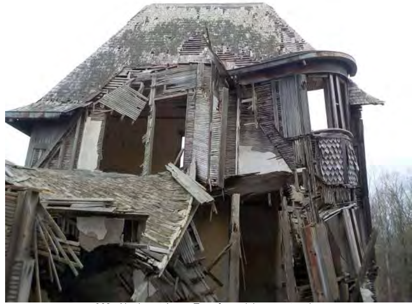
062 - Northeast Area - Top of remaining structure.jpg
