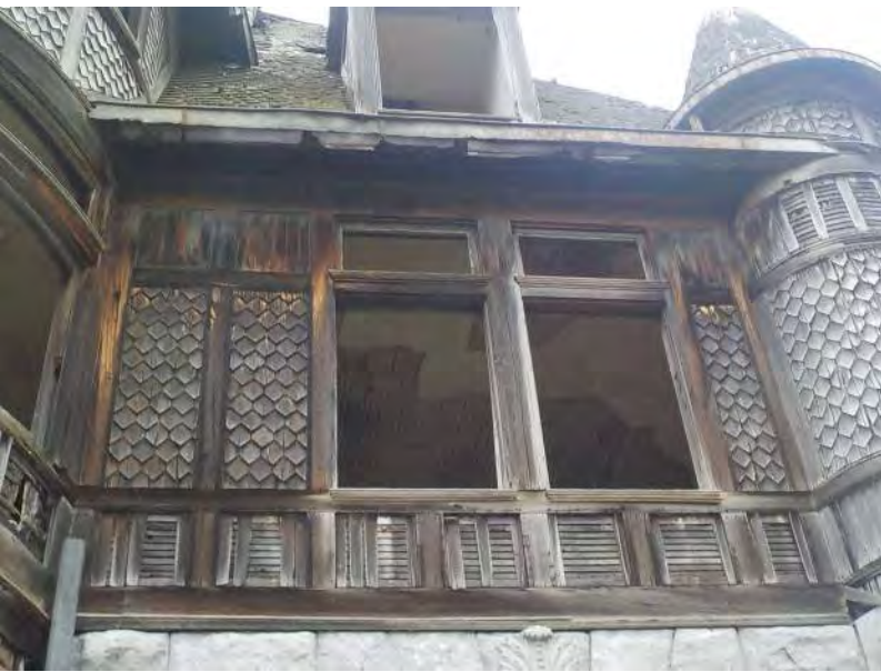
013 - Upper building exterior overview 8.jpg
