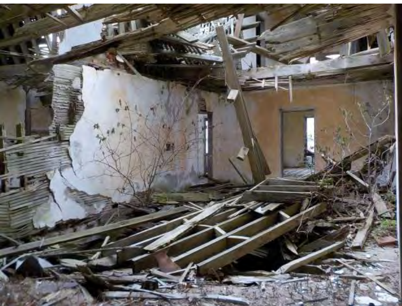
089 - Third Floor - Overview of central area.jpg
