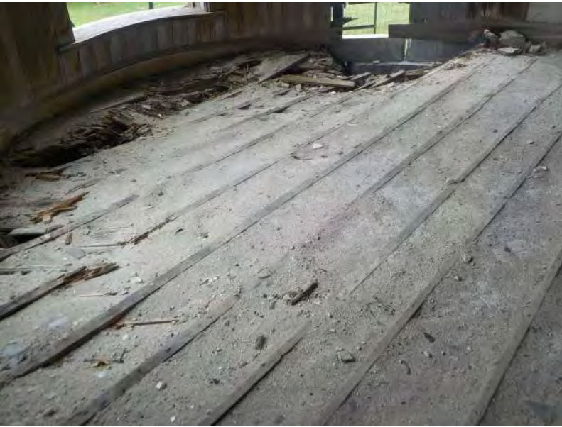
127 - First Floor - Overview of floor 1.jpg
