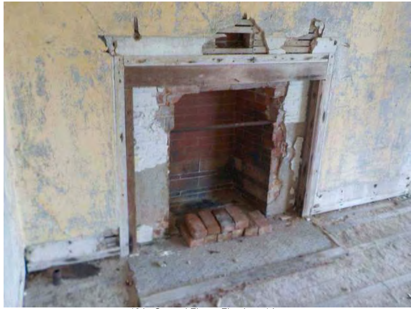
104 - Second Floor - Fireplace 1.jpg
