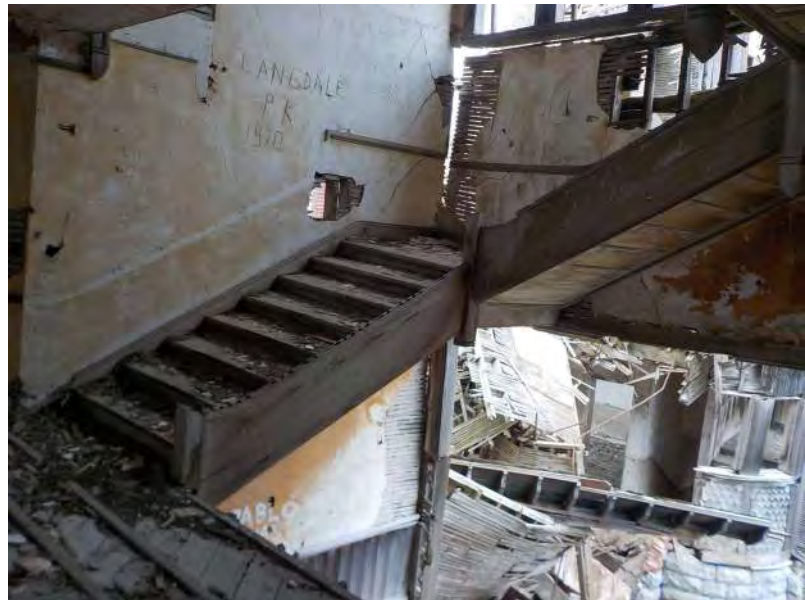
094 - Second Floor - Staircase to 3rd floor 1.jpg
