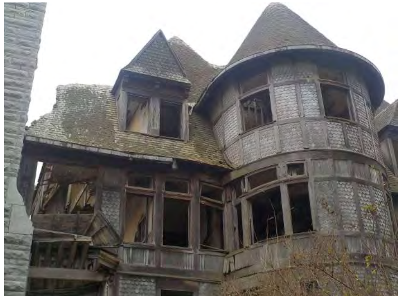
012 - Upper building exterior overview 6.jpg
