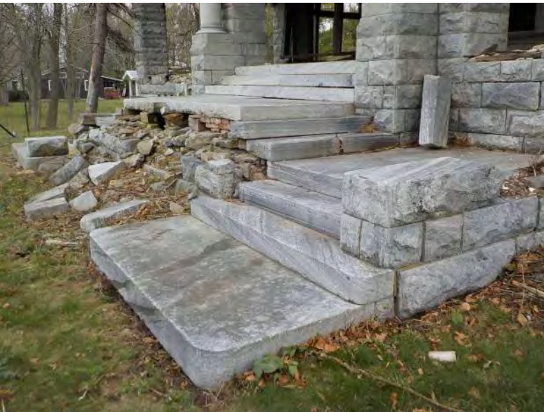
027 - Exterior masonry - SW entrance 3.jpg
