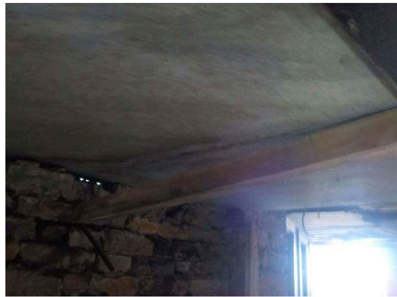
140 - Basement - Supports under stone floor at SE entrance.jpg
