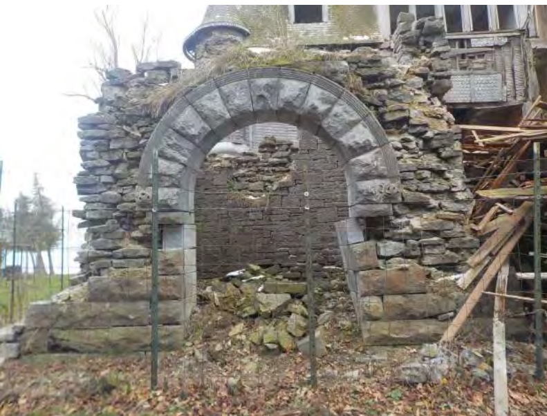
059 - Northeast Area - NE stone arch.jpg
