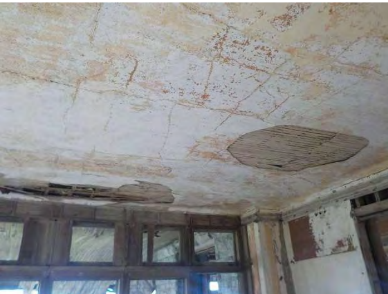
119 - First Floor - Overview of ceiling.jpg
