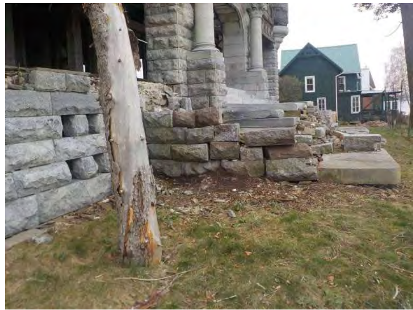
026 - Exterior masonry - SW entrance 2.jpg
