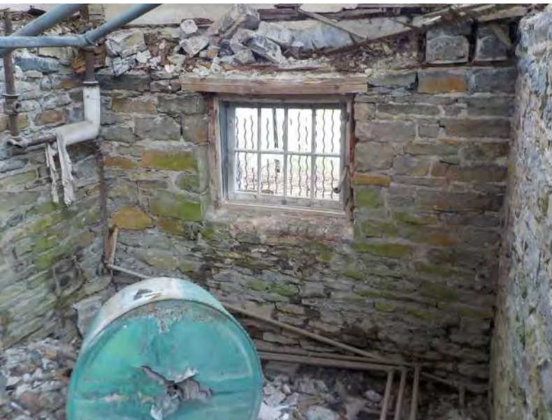
071 - Northeast Area - Basement walls 3.jpg
