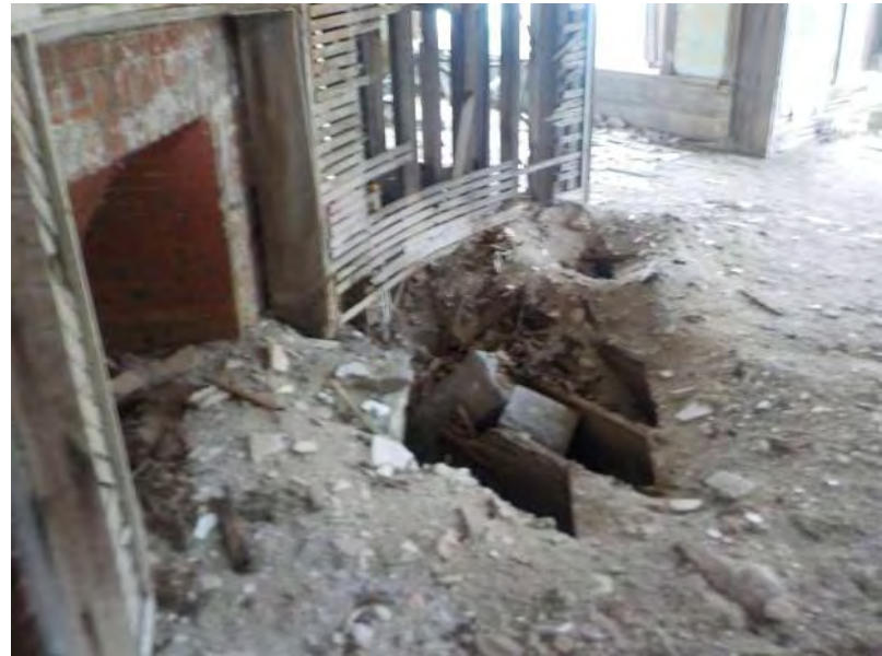
132 - First Floor - Overview of floor 6.jpg
