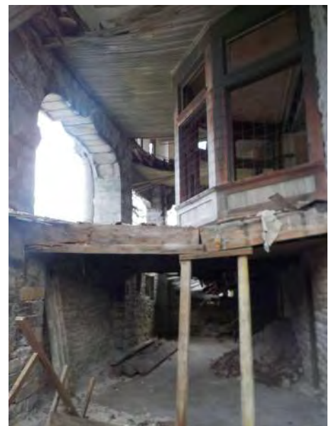
138 - Basement - First floor shoring near south corner.jpg
