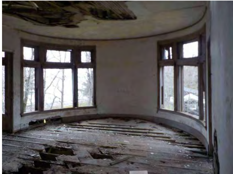
106 - Second Floor - Overview of floor 1.jpg
