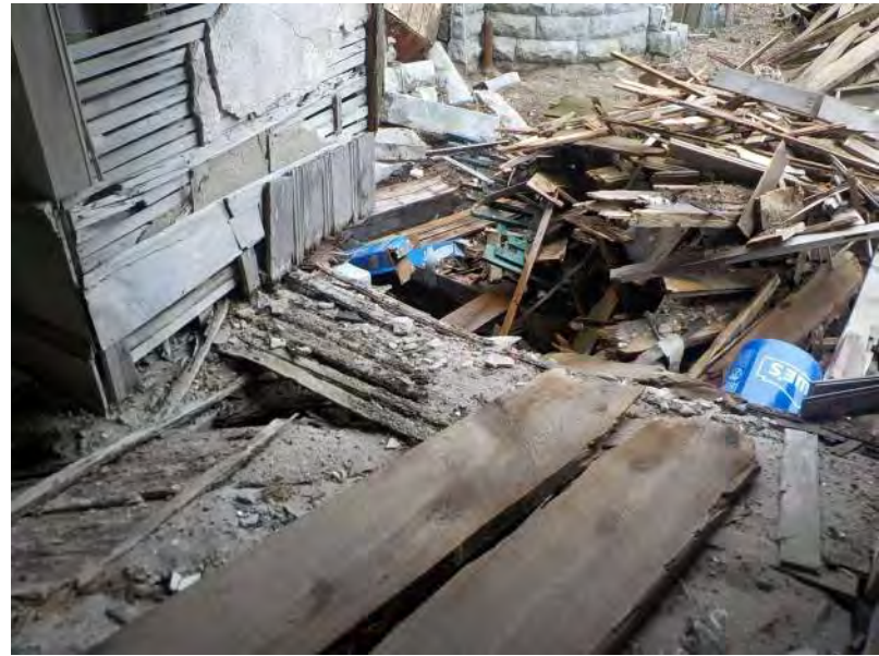
128 - First Floor - Overview of floor 2.jpg
