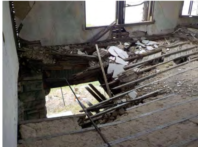
114 - Second Floor - Overview of floor 9.jpg
