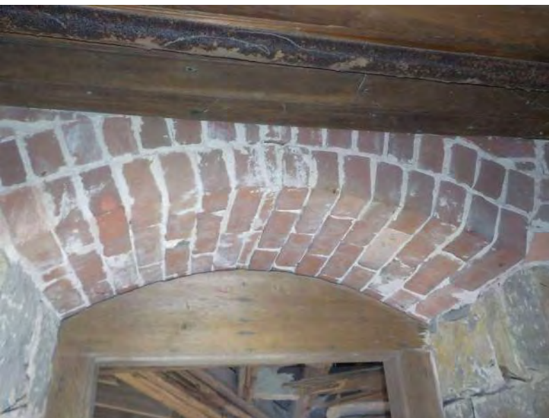
149 - Basement - Arch over opening 4.jpg
