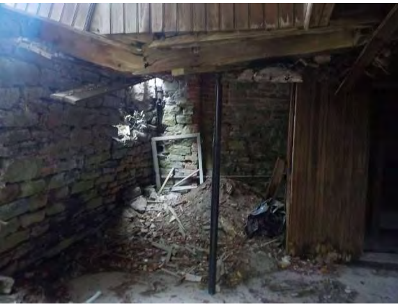
139 - Basement - First floor shoring near stairs.jpg
