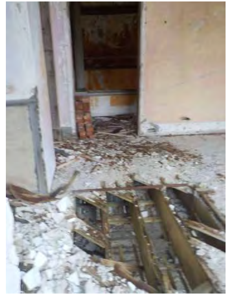
110 - Second Floor - Overview of floor 5.jpg
