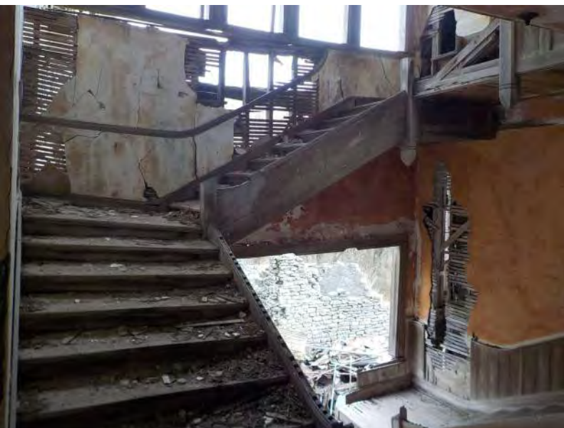
095 - Second Floor - Staircase to 3rd floor 2.jpg
