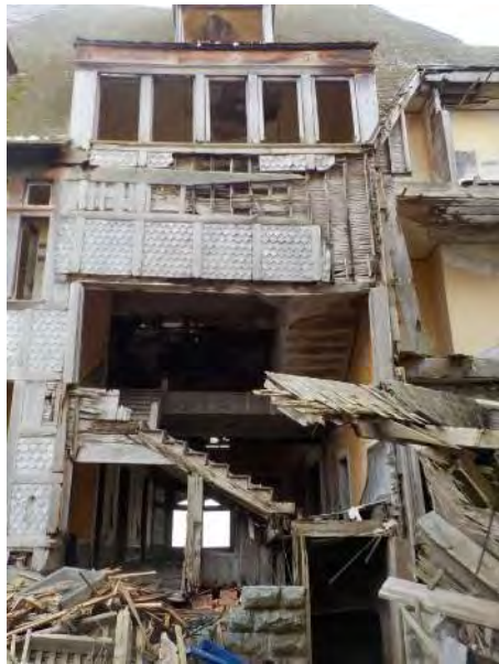
015 - Upper building exterior overview 10.jpg
