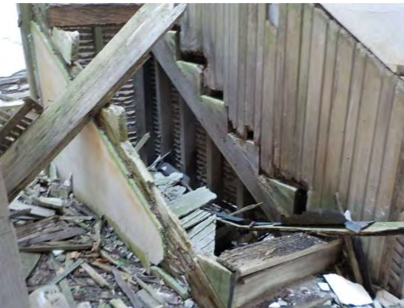
085 - Third Floor - Secondary staircase.jpg
