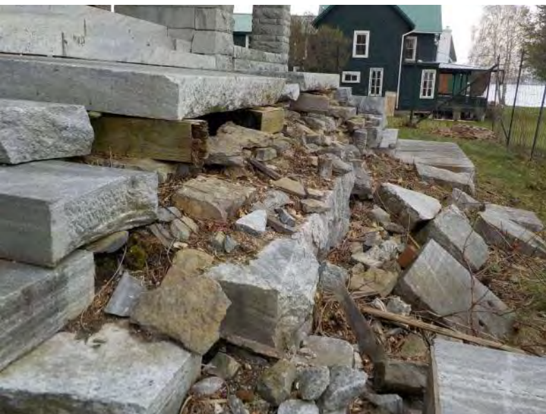
029 - Exterior masonry - SW entrance 5.jpg
