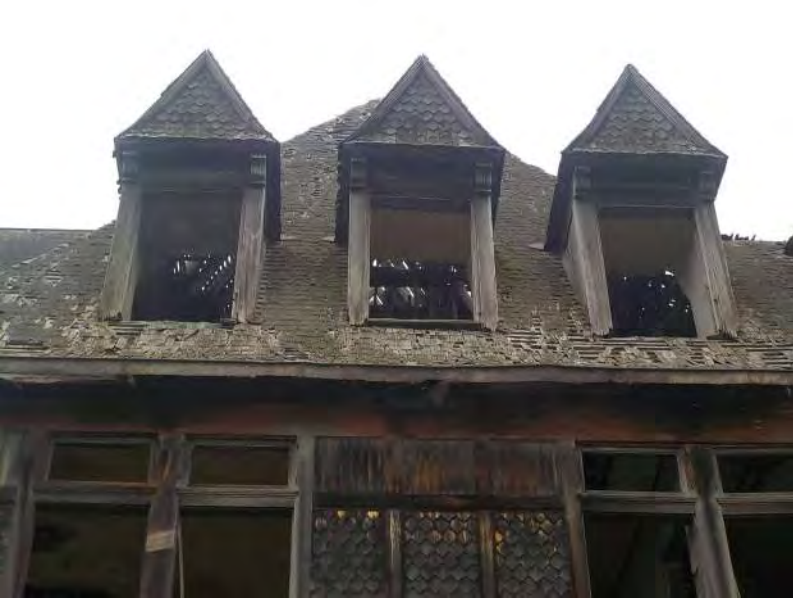
009 - Upper building exterior overview 3.jpg
