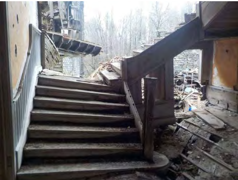
117 - First floor main staircase 2.jpg
