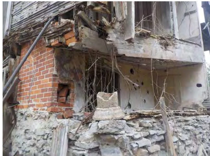
066 - Northeast Area - First floor level overview.jpg
