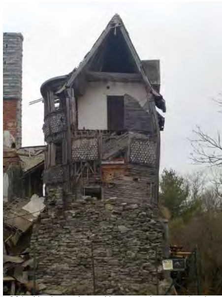
061 - Northeast Area - Upper section overview.jpg
