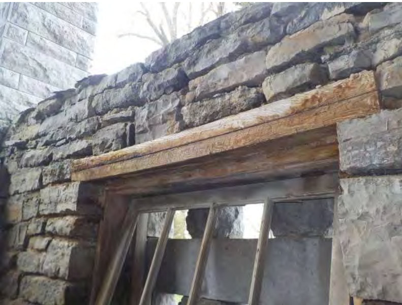
153 - Basement - Wood plank lintel over opening 2.jpg
