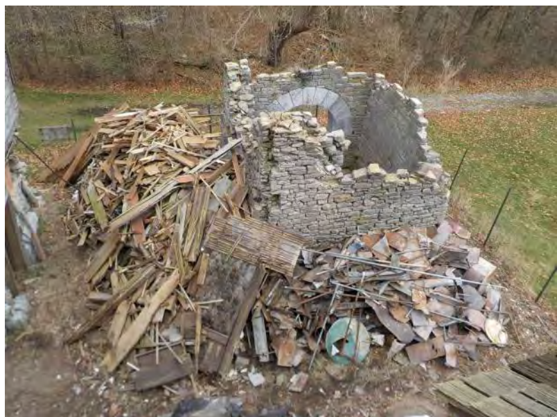
058 - Northeast Area - Base of tower.jpg
