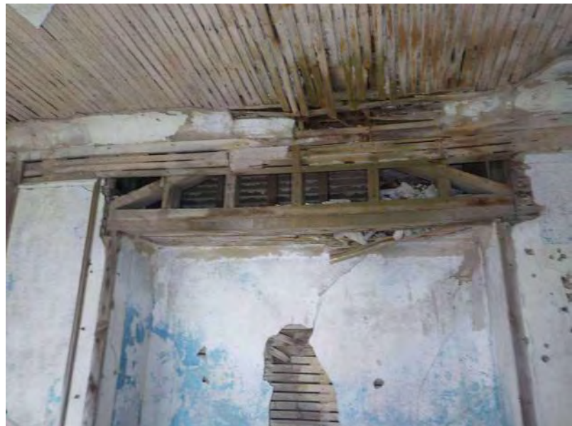
120 - First Floor - Wall opening header 1.jpg
